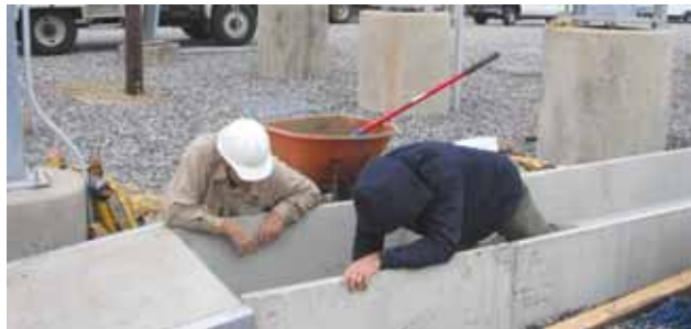
Top: CHEC Lineman Kerry Hooper wires new regulators for new circuits out of the Waves substation.
